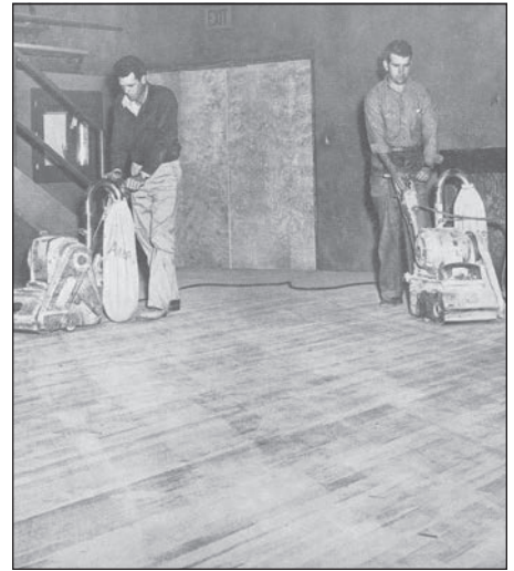
Workmen from Salinas Valley Floor Company, owned by Ray Pool, sanding the gym floor.
